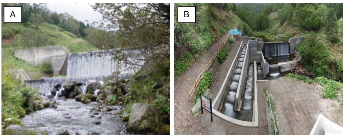
Fig. 4 Check dam before and after modification by installation of a fishway
