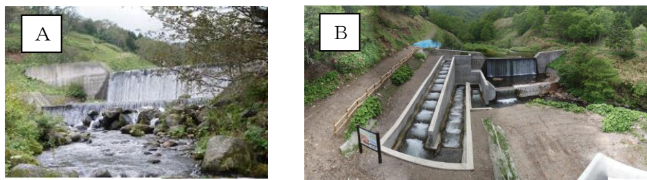
Fig. 4 Before and after dam modification (installation of new fishways)
